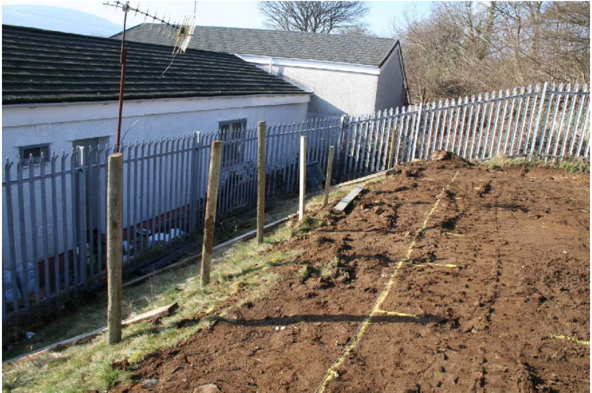
So the site was cleared and timber raised beds were erected making planting a joy for the young people and weeding a doddle.
