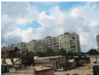
Intensive urbanisation in the 19th century when the demand for concentrated labour increased significantly
