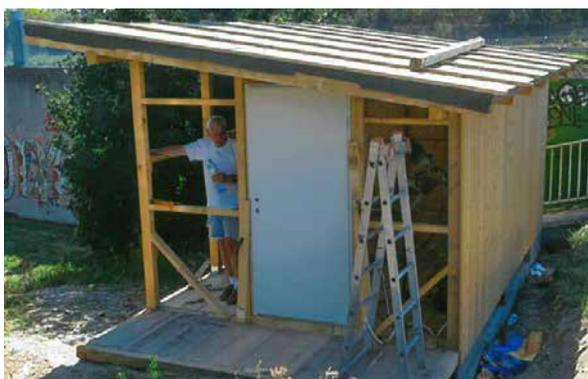
*The roof sealing with bitumen sheets and the front door were next, ...*
