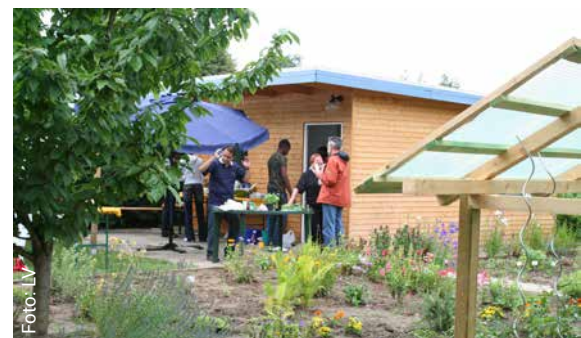
Shed and garden after their renovation.
