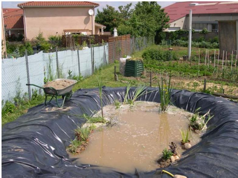
Once the perimeter of your pond is mapped out, it is time to roll up your sleeves and take the pickaxe, spade and shovel to dig the hole. The earth dug out of the hole can be put on the bank: that way you will have less to dig. If you add a depth of 20cm of levelling soil on the bank, you will only have 40cm to dig to achieve a pond 60cm deep.
