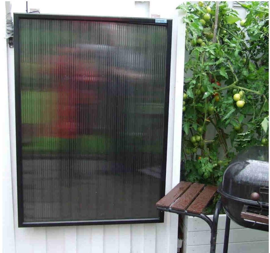
Solar collectors provide ventilation and prevent humidity in many Scandinavian allotment houses – an example from Stockholm – Sweden.
